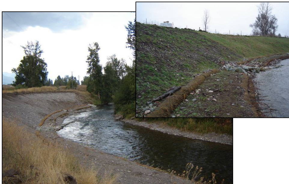
Figure A-1. Photograph of coir logs immediately after installation along the toe of an eroding slope and eight months after installation (inset). Plant material was not incorporated into the coir logs at this project site.
