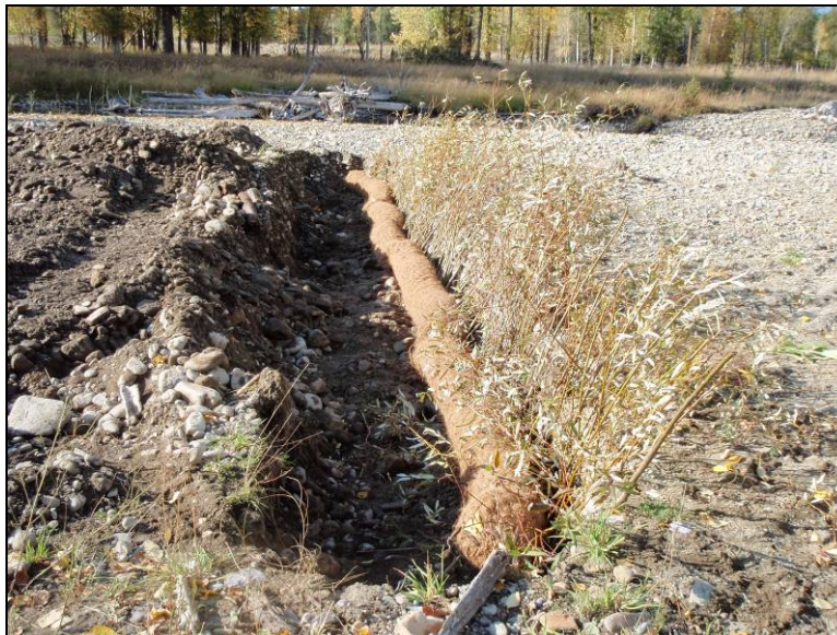
Figure A-2. Photograph of buried coir log fascine floodplain treatment during construction.
