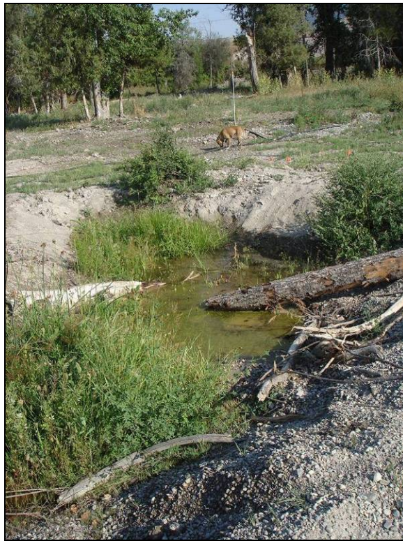
Figure A-4. Photograph of constructed floodplain swale five months after construction.
