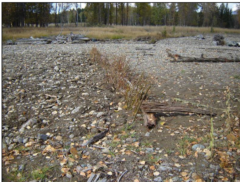
Figure A-3. Photograph of buried coir log fascine floodplain treatment immediately after construction.
