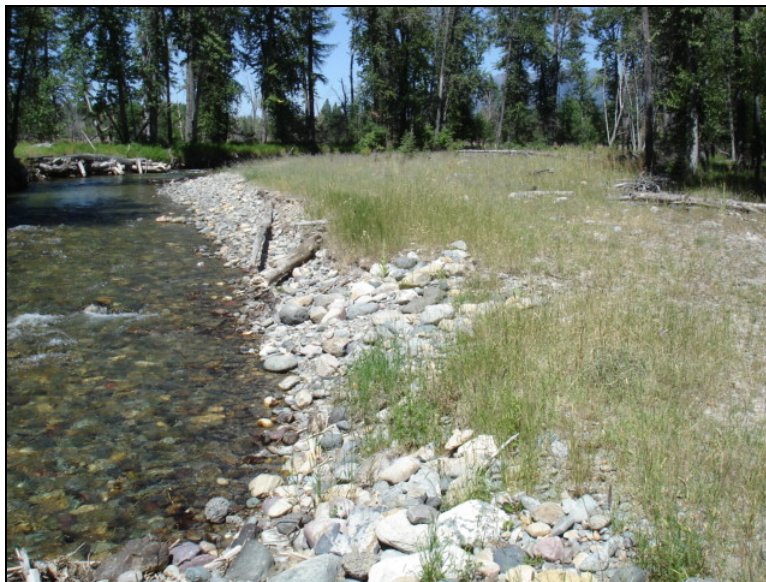
Figure 8. Photograph of existing conditions within the Demo reach, where banks lack mature riparian vegetation. During initial channel construction in 2001, concerns of possible avulsions or headcutting resulted in the construction of floodplain surfaces that are uniform and at elevations that are less frequently accessed by high flows.
